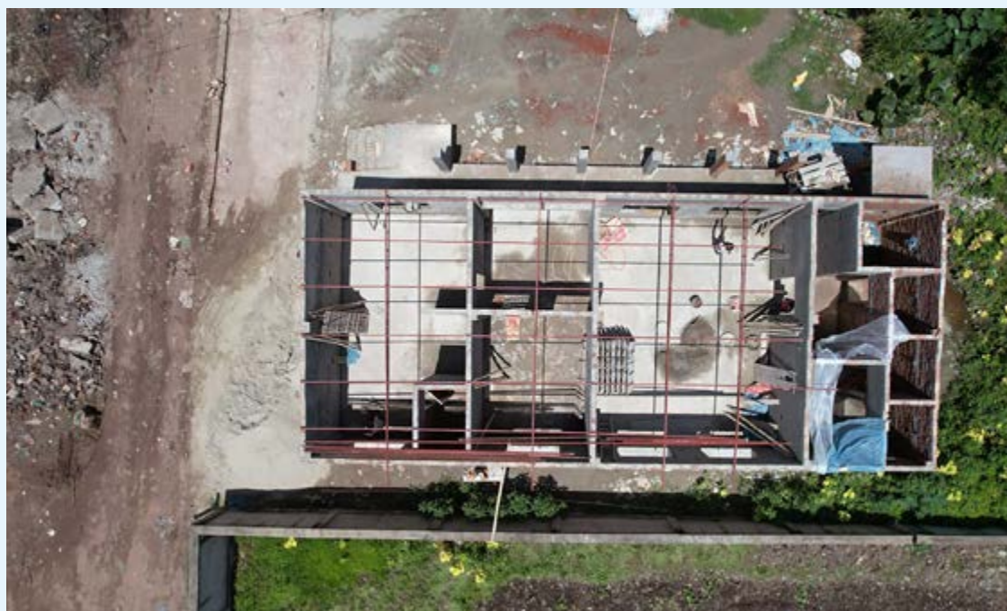
Figure 47: Sanitation facilities under construction at the Rajbandh site. Photo by Saptarshi Mondal, 2024.
