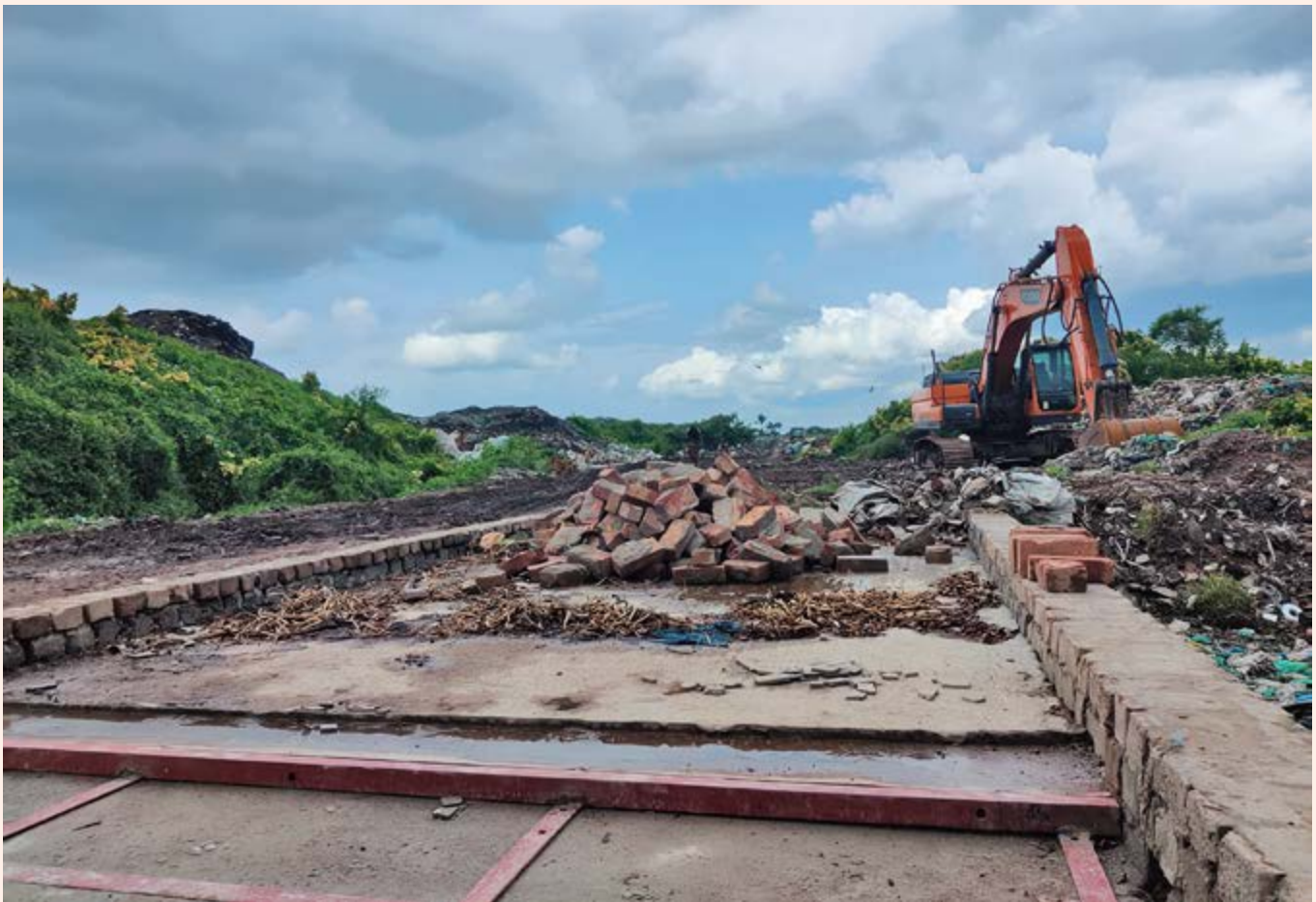
Figure 54: Weighing station under construction (final curing). Photo by Sourav Saha, 2024.
