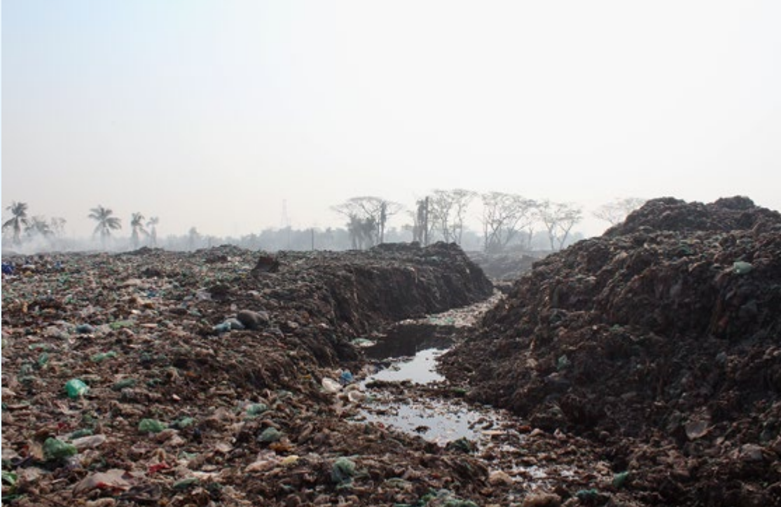
Figure 38: Drainage line excavated on top of the waste pile. Photo by Senta Berner, 2023.
