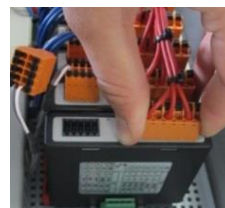
Fig. 12: Installing the controller module (similar to picture)
